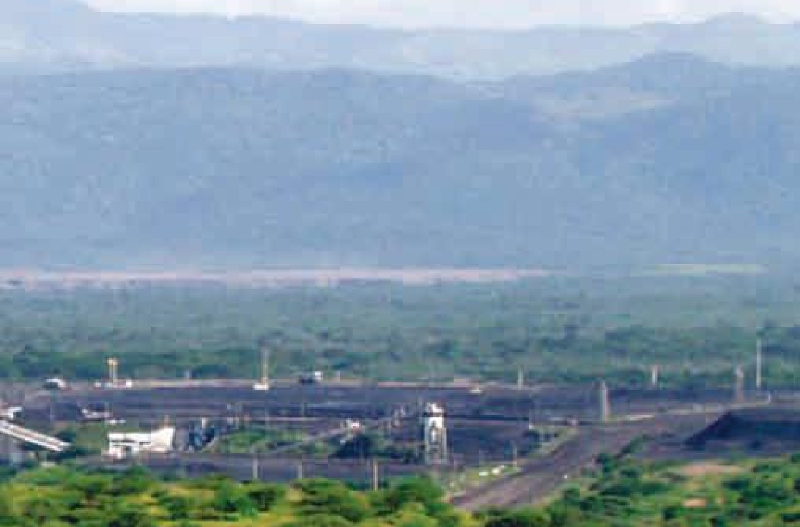
Silos coal collection centre
