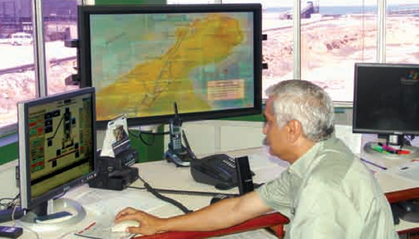
Coal Handling Control Centre in Puerto Bolívar
