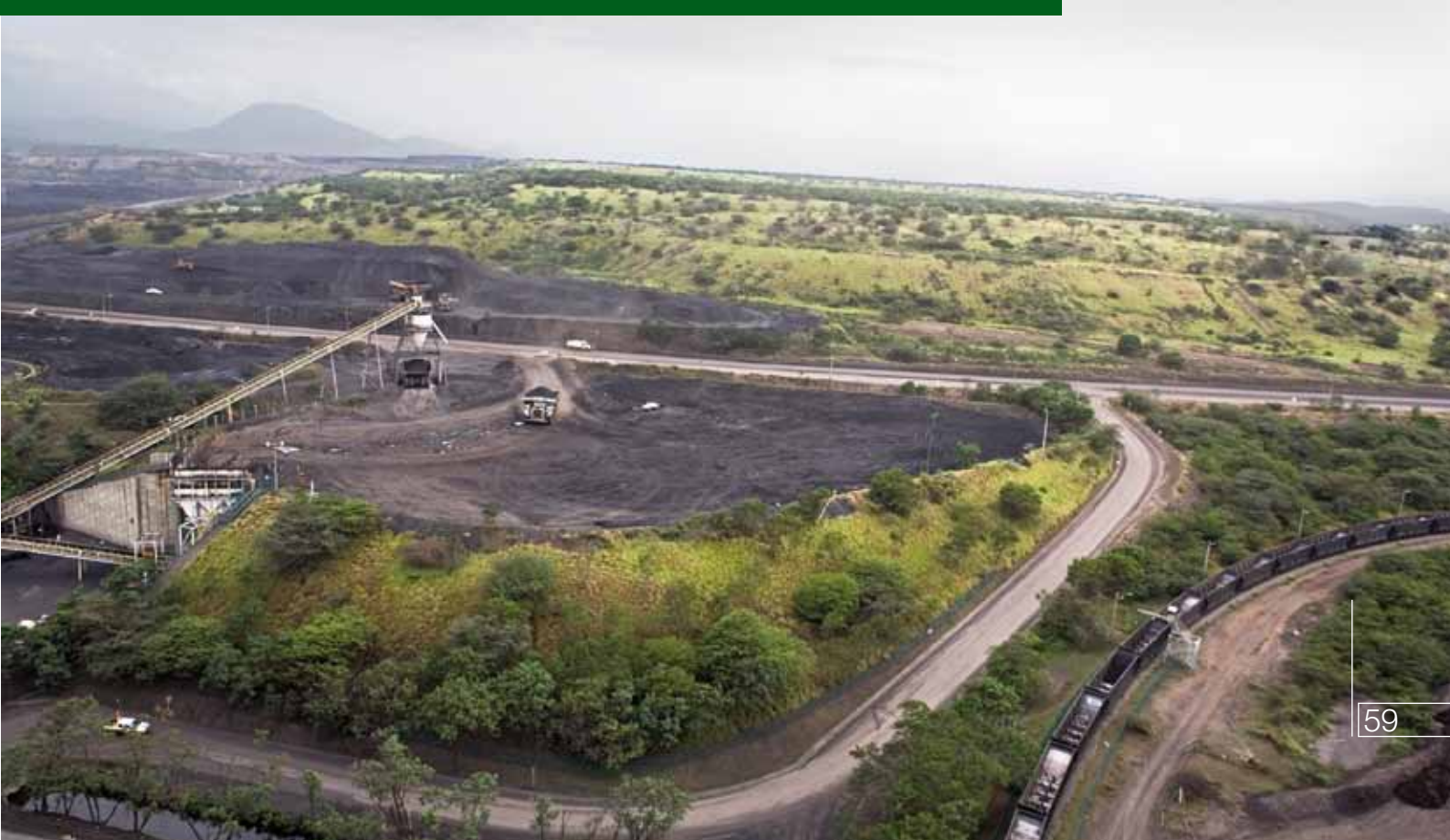
Land reclamation in an integrated process of coal haulage, crushing plant, and rail transport at Cerrejón
