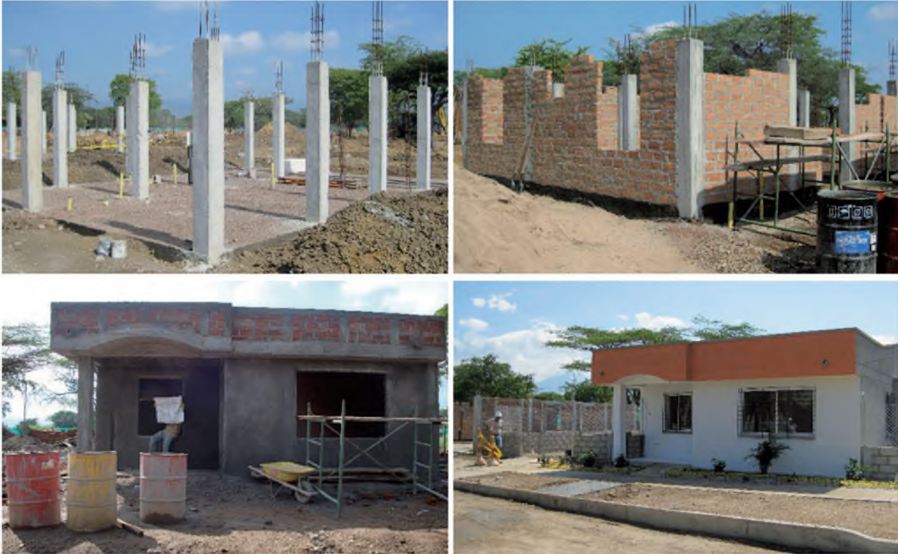
Construction of housing in Roche.
