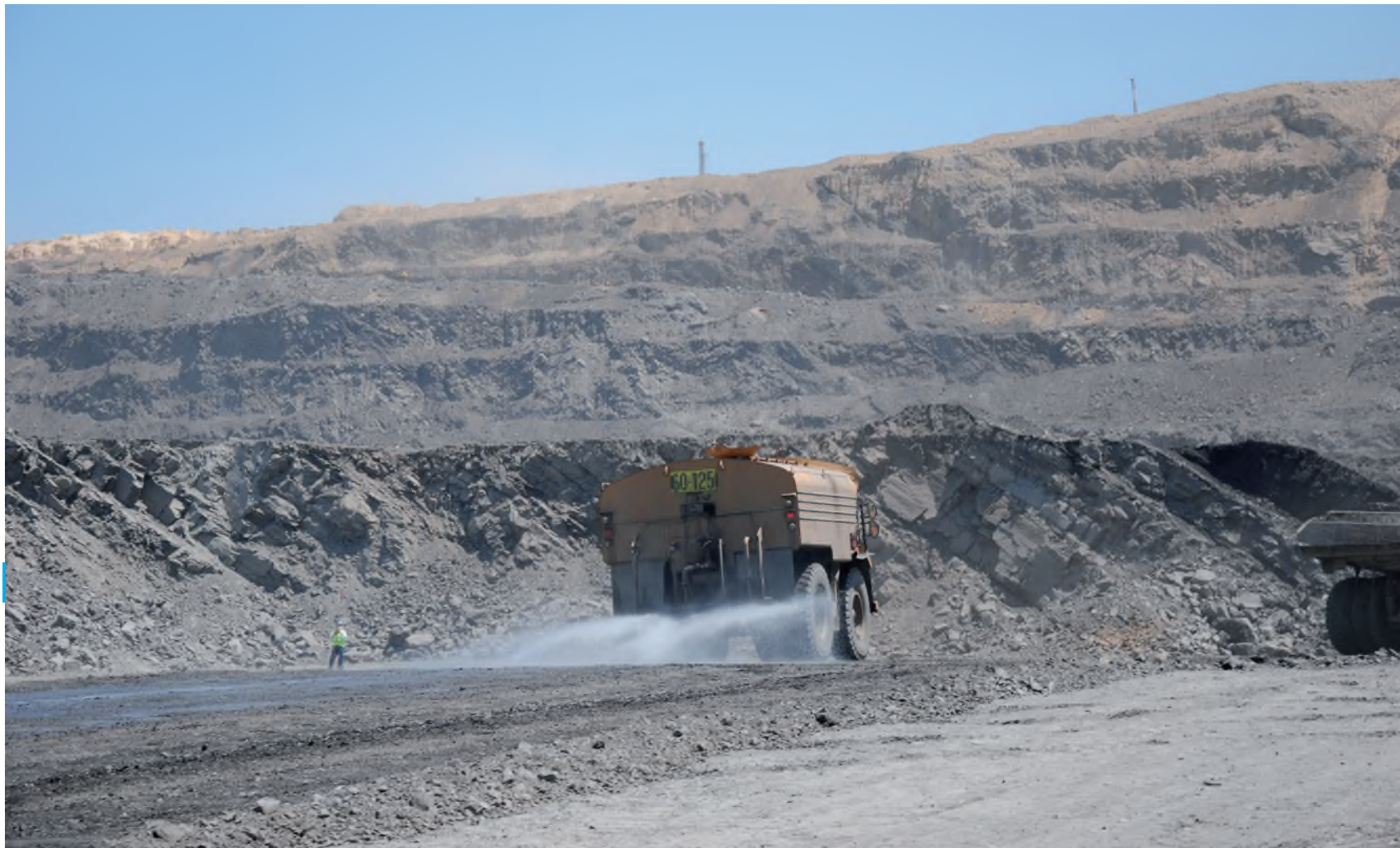
Water tanker spraying for dust control on haulage roads.
