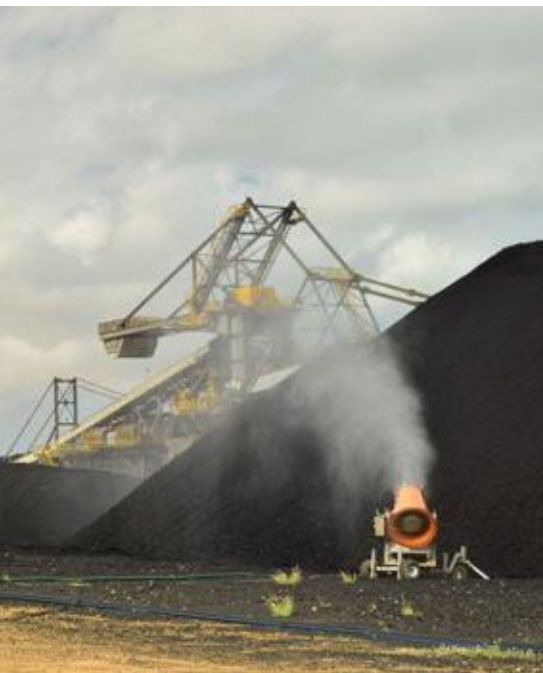
■ Fog canons and sprinkler systems.
